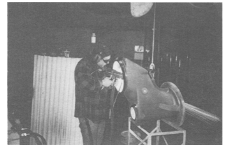
Fig. 4 95MXC repair of pump housing
